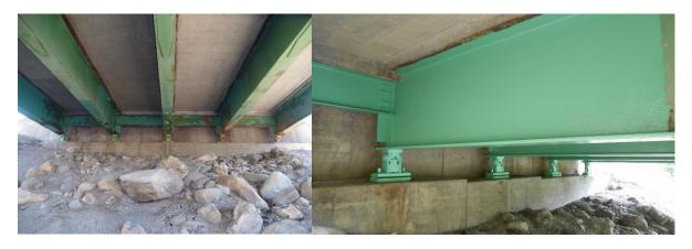
Oil Beam Ends and Bearings
